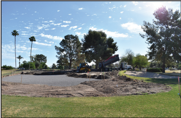
USGA Greensmix being placed on hole 17 green
