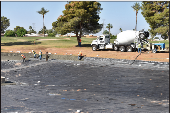
Lake Liner and shoreline being installed
