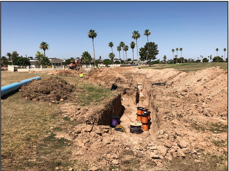
Connection of mainline from Willowcreek and Willowbrook will allow either golf course to be watered from either pump station
