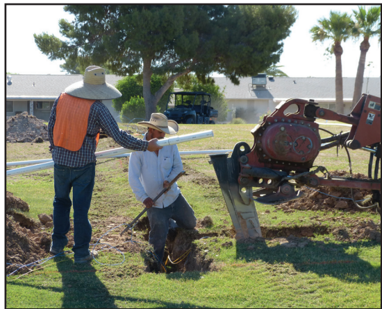
Above: Irrigation lateral being hooked up to vibratory plow Right: New irrigation pump station
