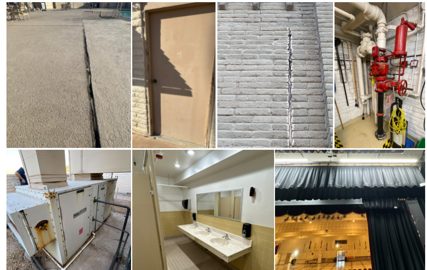
Figures Above - Selection of Facility Condition Assessment Areas
